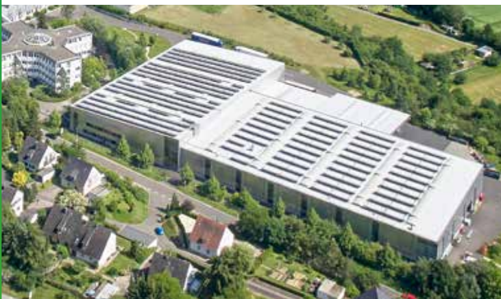
BITO Meisenheim - Photovoltaic panels on plant roof
