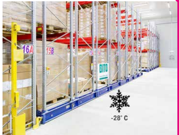
Mobile pallet racking in a cold store
