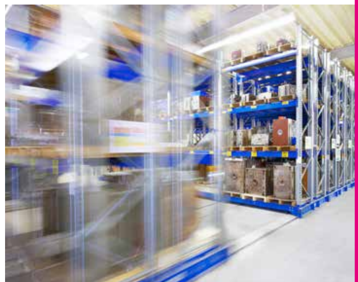
Mobile pallet racking facility
