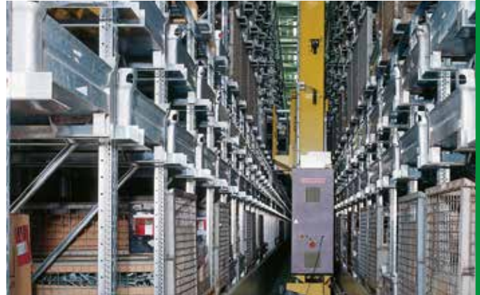
Automated pallet live storage facility with single position storage
